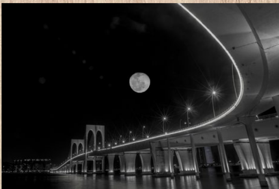
Ponte de Sai Van 02 WING HO CHAN, Hong Kong
